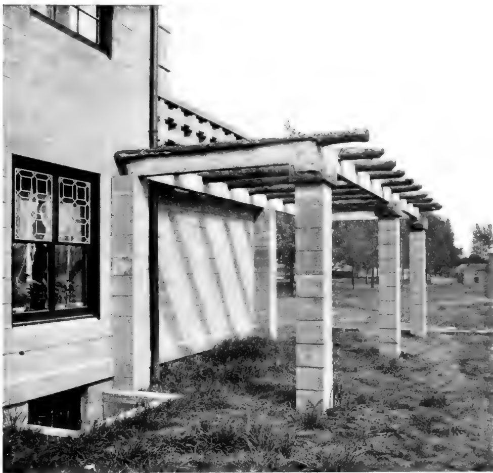
15—Leaded Glass Windows and a Pergola Lend Character to the Building
